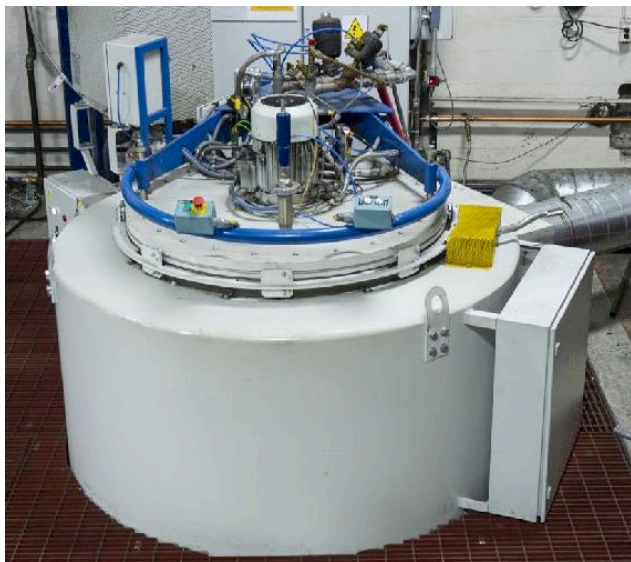
TEMPER AND NITRIDING FURNACE
