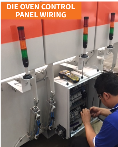
DIE OVENS ASSEMBLY - INSULATION, ELECTRICAL & TESTING
